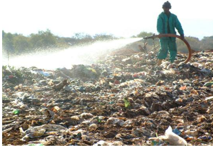
Figure 7 Watering the crushed waste
