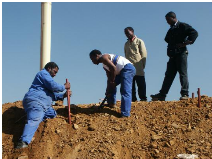
Figure 12 Hammering pipes into windrow
