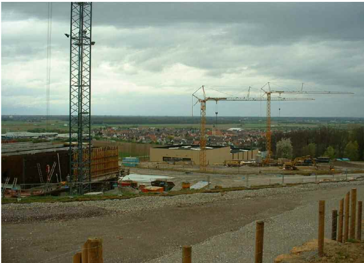
Figure 11 Construction of the Percolators (left) and Land Scaping, February 2005
