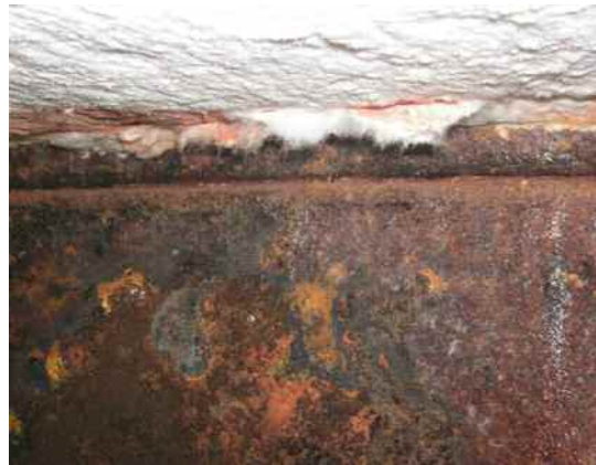
d) Wall of combustion chamber (inside)
