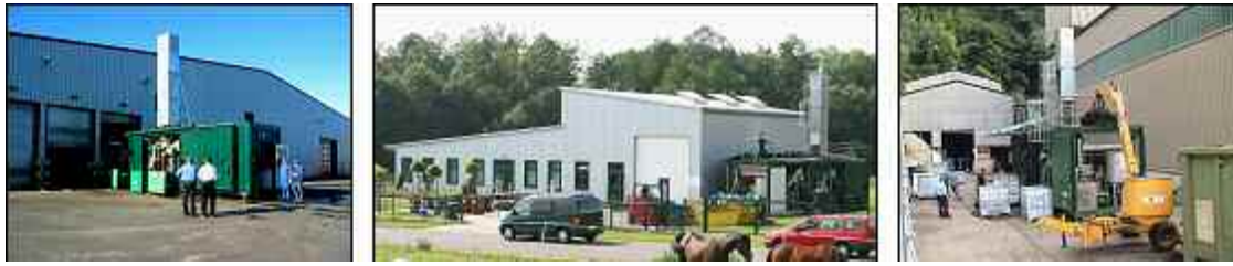
Figure 2: Different locations of the SCHUBIO®-Demonstration Plant
