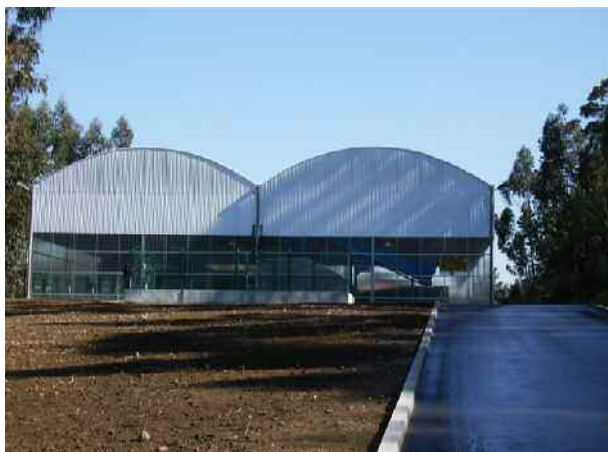
Figure 1 View of the vermicomposting unit
