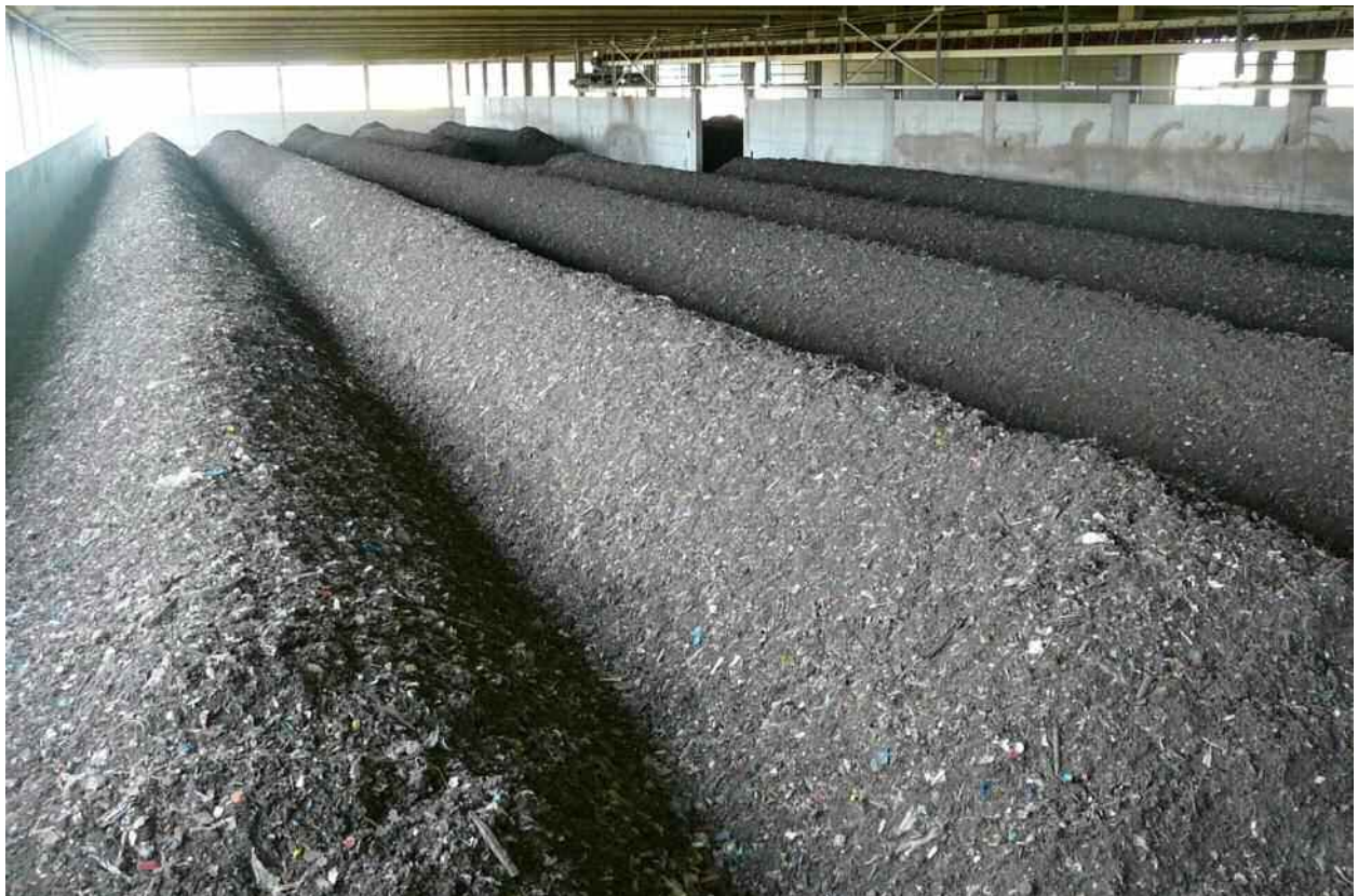
Figure 2: Maturation MBT Rosenow after reorganisation towards windrows
