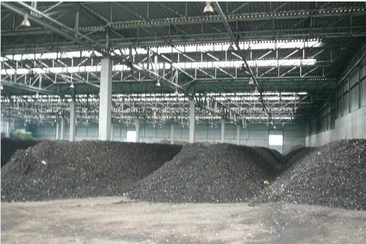
Figure 1: Maturation MBT Cröbern after changing to windrows
